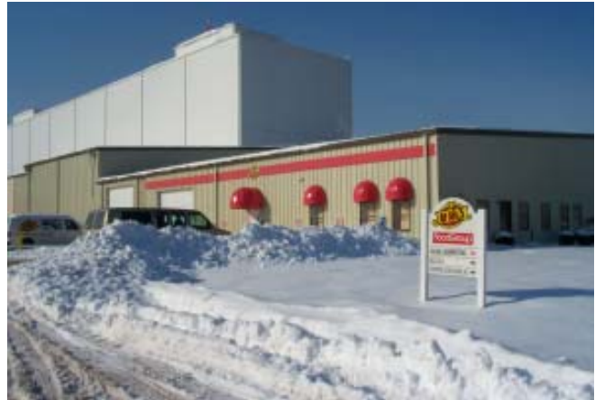
JTM Cafe and new high rise automated storage freezer. This is the building you want. Park anywhere in the parking lot area and then come to the cafe. Our tour will start there. Hopefully all of the snow will be melted by then.
